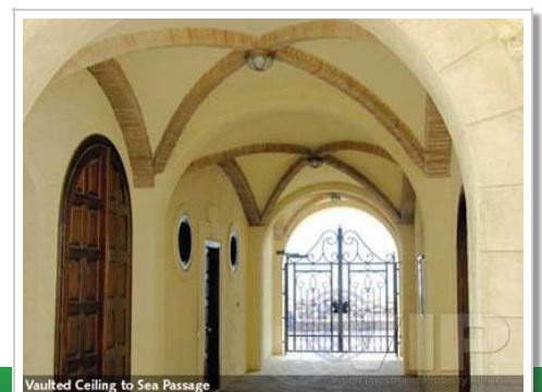
Vaulted Ceiling to Sea Passage
